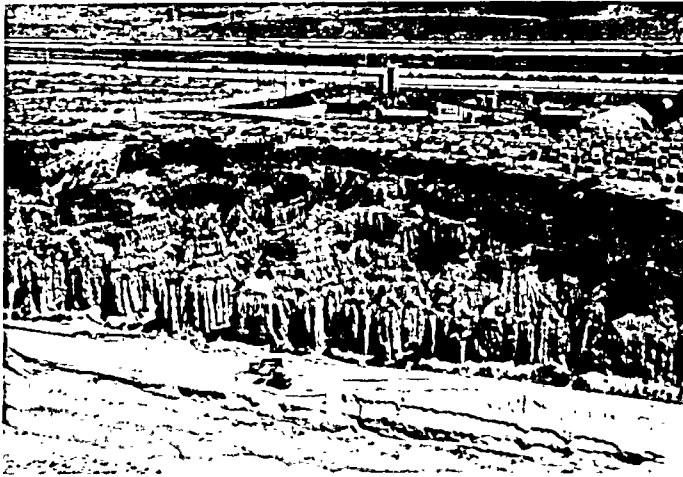
NRR site visit team members investigate barranca (sea cliff) near the San Onofre nuclear generating station units 2 and 3. The San Onofre plant will be required to help divert nearby highway water run-off to protect the barranca formation, which is endangered because of erosion of unconsolidated sandstone.
