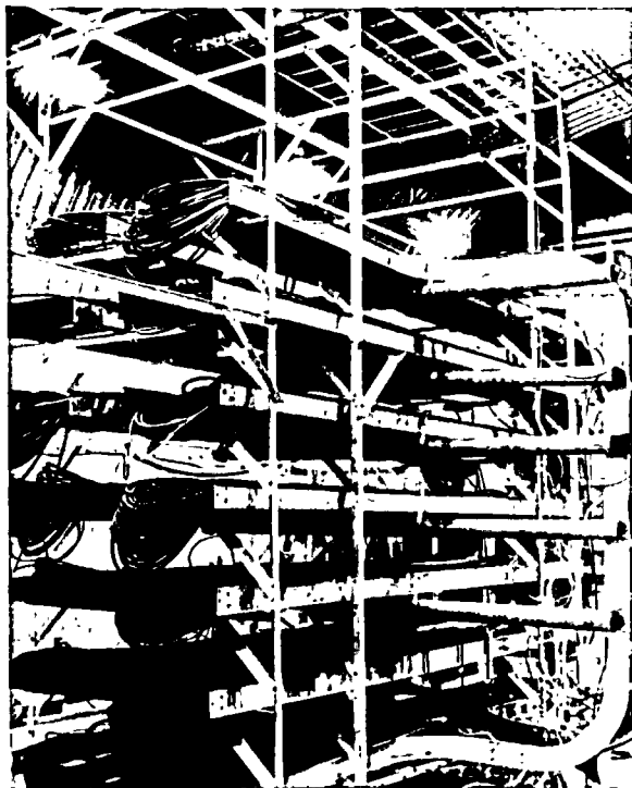
Stacked cable trays are tested at Sandia Laboratories, New Mexico, to assess the degree of protection afforded by the vertical and horizontal separation of safety divisions. The cable tray at the very top of the photo represents the vertical safety division separation being tested.
