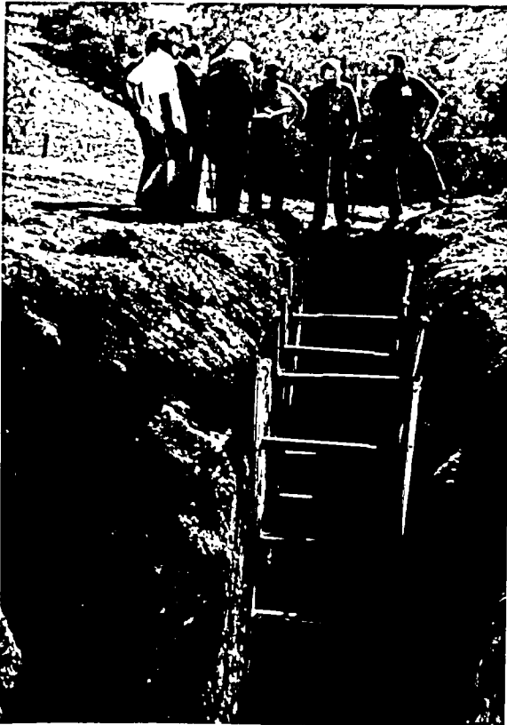
Geological and seismological experts from NRC's Office of Nuclear Reactor Regulation, the U.S. Geological Survey, the California Division of Mines and Geology, and Earth Sciences Associates examine trenches at the General Electric Company's Vallecitos Nuclear Center near Pleasanton, California, for evidence of geologic faulting. This investigation in October 1977 led the NRC staff to order the General Electric Test Reactor shut down on October 27, 1977.
