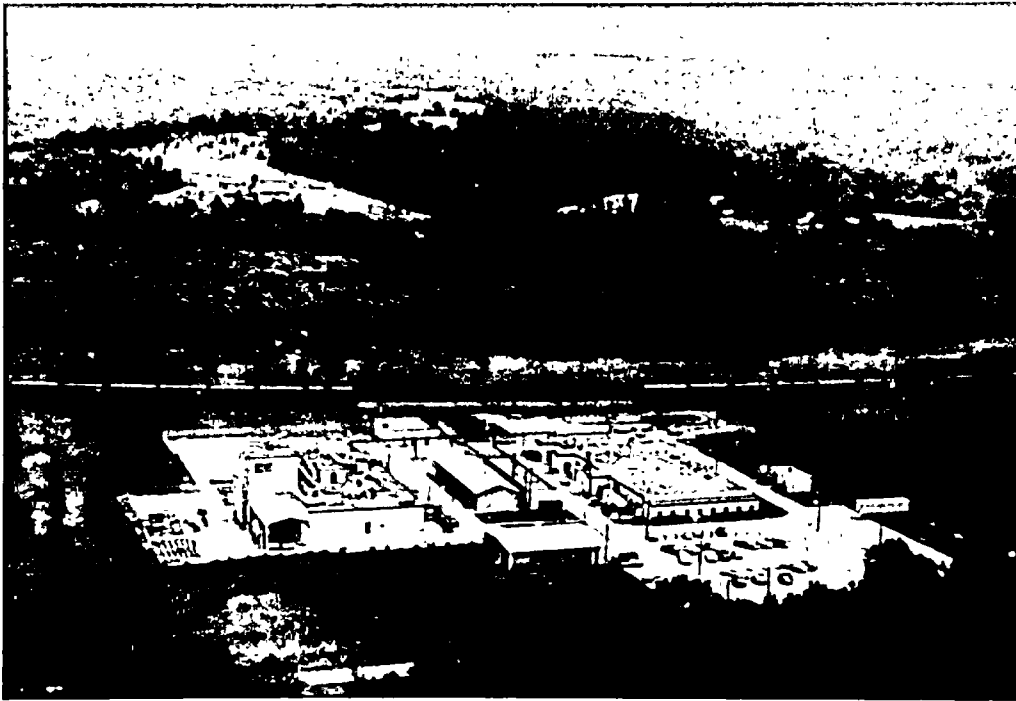
This is Combustion Engineering's Hematite, Missouri, uranium fuel fabrication plant. Operations include conversion of low enriched UF_4 to UO_2 , fabrication of UO_2 pellets, and related processes. Finished pellets are shipped to Combustion's Windsor, Connecticut, facility to be used in the manufacture of fuel elements for power reactors.
