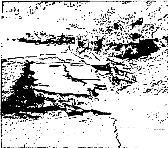
NRC develops standards for assessing geologic hazards such as earthquakes and faulting. The photograph at the left shows damage to a highway due to high vibratory ground motion from the 1959 Hebgen Lake, Montana, earthquake. A fault scarp of about 15 feet produced during the same earthquake is shown at right.
